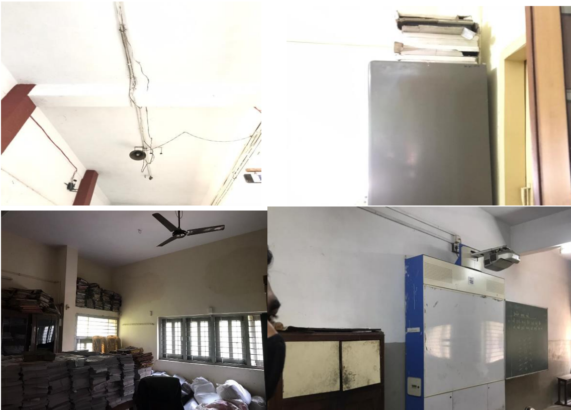
Figure 5: Common structural and non-structural risks in school building
